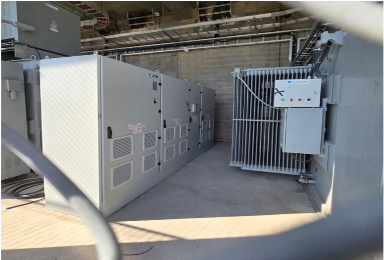
Figure 22 Photos of installation
