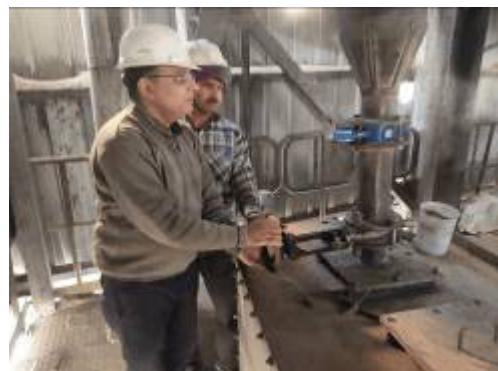
Figure 11 Installation of feeding system for Oxy-booster
