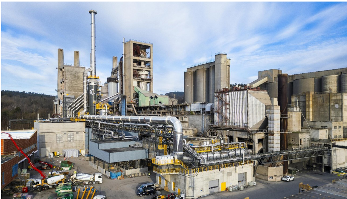
Figure 10: Norcem cement plant at Brevik, Norway, integrated with carbon capture facilities.
