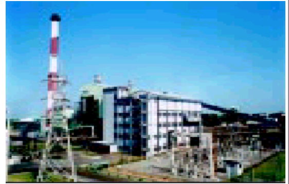
Commercial co-generation plant
