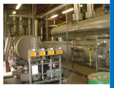
in a vaporizer. In this vaporizer, the working liquid is converted to vapour. This vapour is utilized to rotate a turbine. The spent vapour is cooled in an air-cooled condenser and the liquid is again fed back to the cycle to pick-up further heat from the vaporizer.
