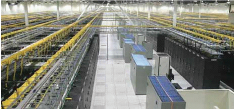
Layout of the overhead cable arrangement
